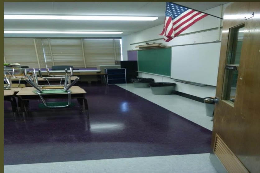
Flooring Replacements at Parkway ES
